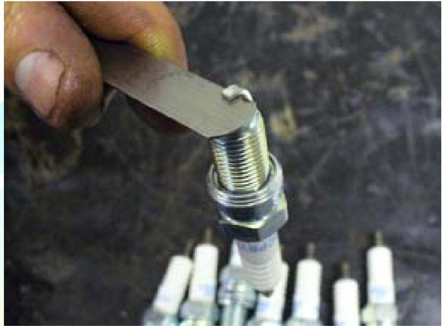
Figure 33: Checking plug gaps before installation
